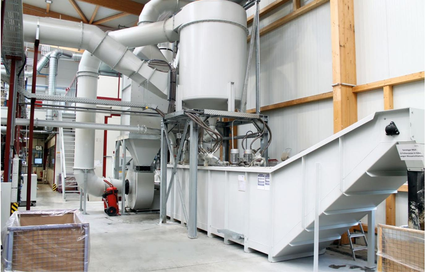
At the extruders, adhesive gases escape as well as dust. This challenging air cleaning task is solved with the VDN-TA wet separator, which improves air quality at the extruders and inside the plant.
